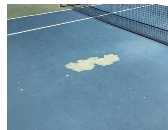
Tennis court surface delamination
