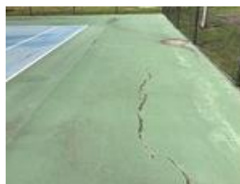
Tennis court surface cracking
