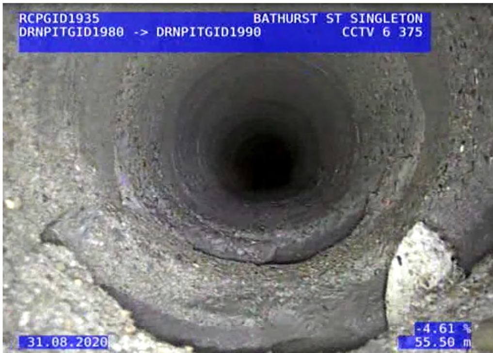
Figure 7.1 CCTV inspection of a stormwater pipe in Bathurst St, note pieces missing from bottom of pipe.
