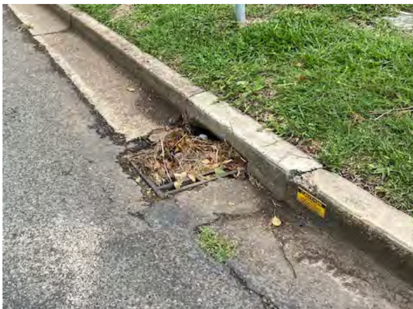
Figure 7.2 Short length inlet pit in 'old' part of Singleton is easily blocked by leaf litter
