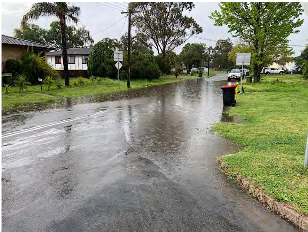
Figure 4.1 Temporary flooding of an urban street in south Singleton after modest rain due to drainage capacity problem, most likely due to blockage (September 2020)
